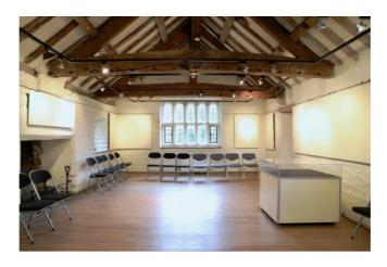
Mortices cut into the tie-beams took smaller timbers that formerly supported a plastered ceiling. First (northernmost) tie-beam far face shows Roman numerals that number the mortices in sequence.
